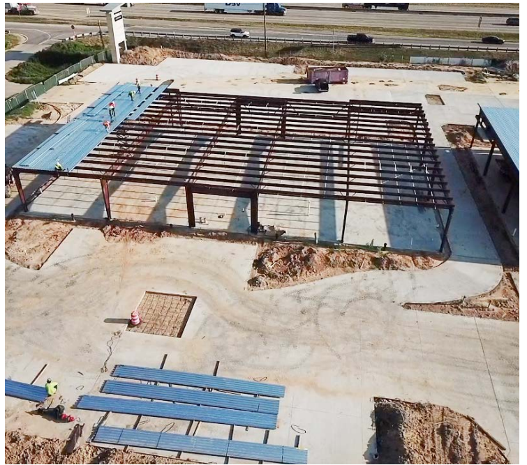
Construction Progression Aug 2024
