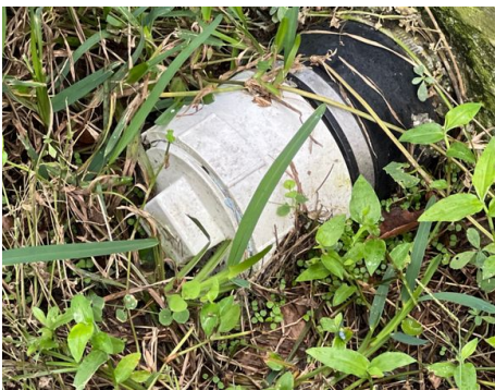
Main Cleanout: Cleanout Location Left Exterior
