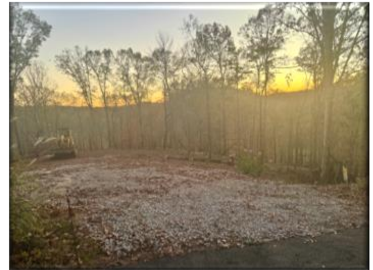
North side of Parcel Construction Site
