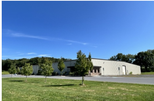
EXISTING PARK FACILITY
