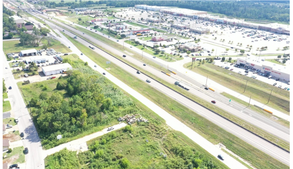
Facing South Along I-45
