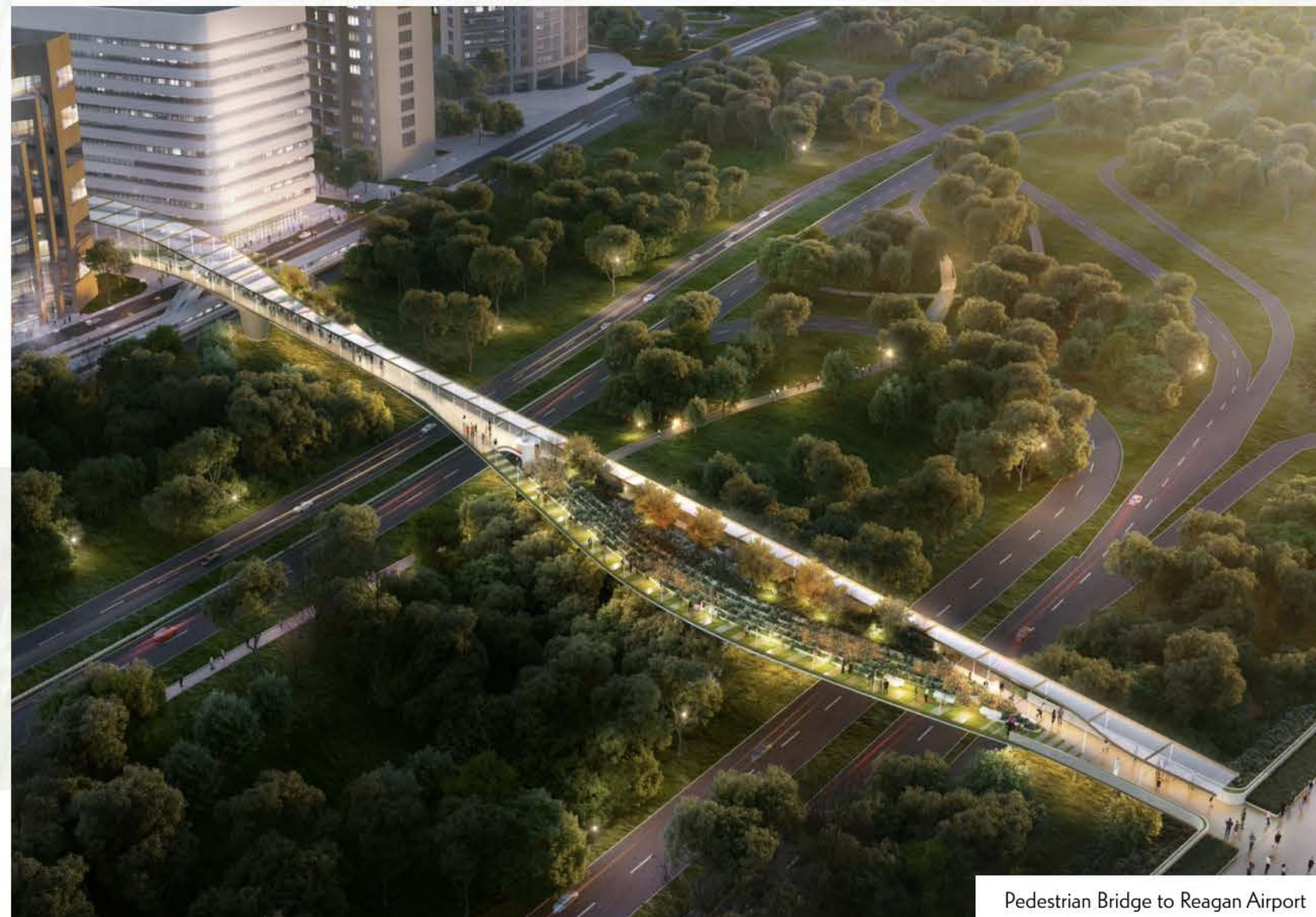
Pedestrian Bridge to Reagan Airport
