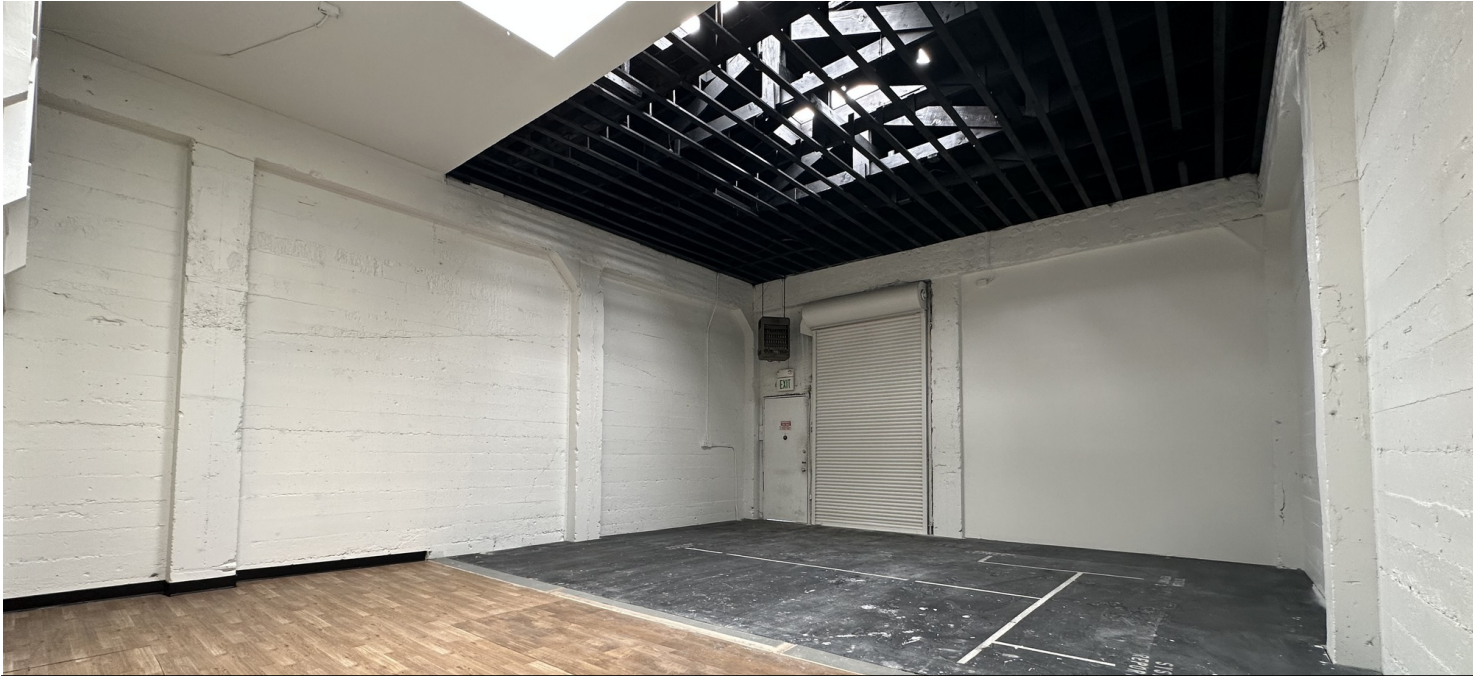
Rear of Building/Production/Shipping & Receiving
