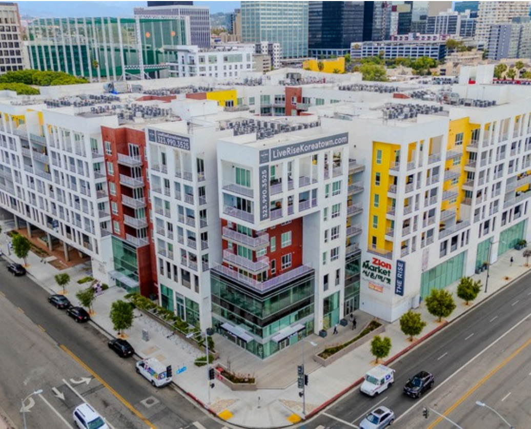
EXTERIOR VIEW FROM OXFORD AVE & 8TH ST
