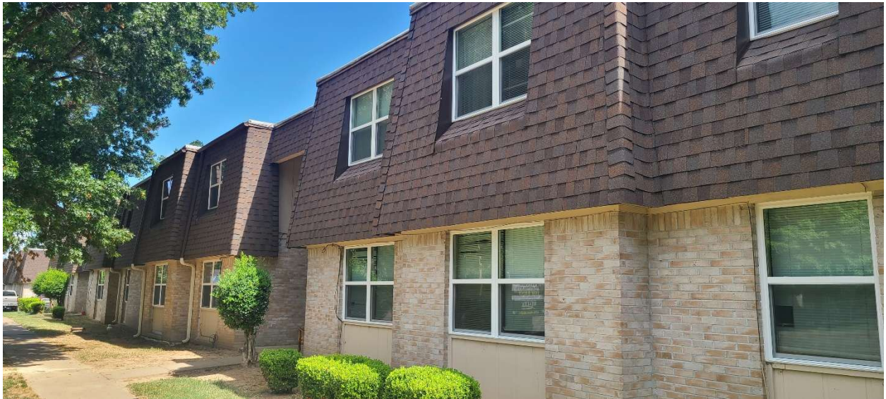
266 Windows were installed in July and August 2024. 50-year Roof Shingles installed in Dec. 2023.
