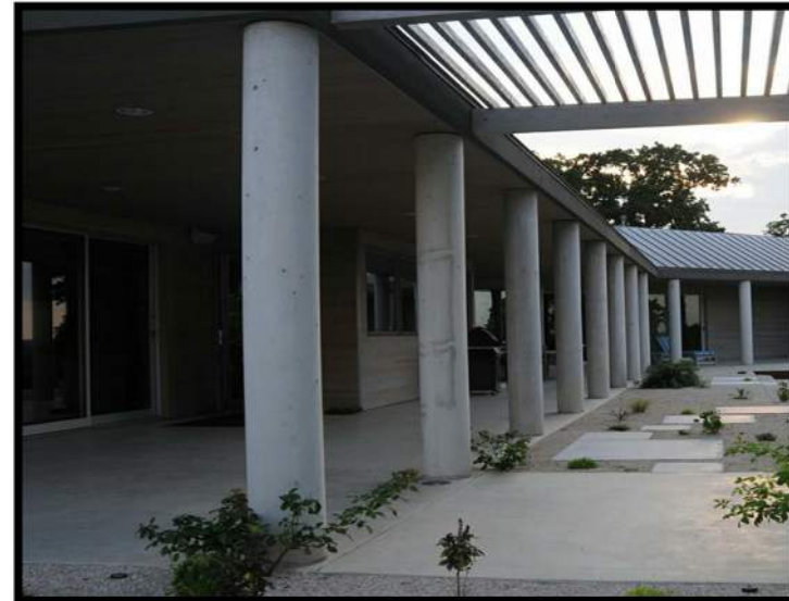
④ CONCRETE COLUMNS
