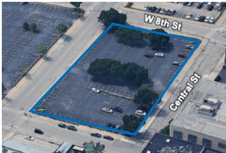
700 WYANDOTTE STREET AND 701 CENTRAL STREET
