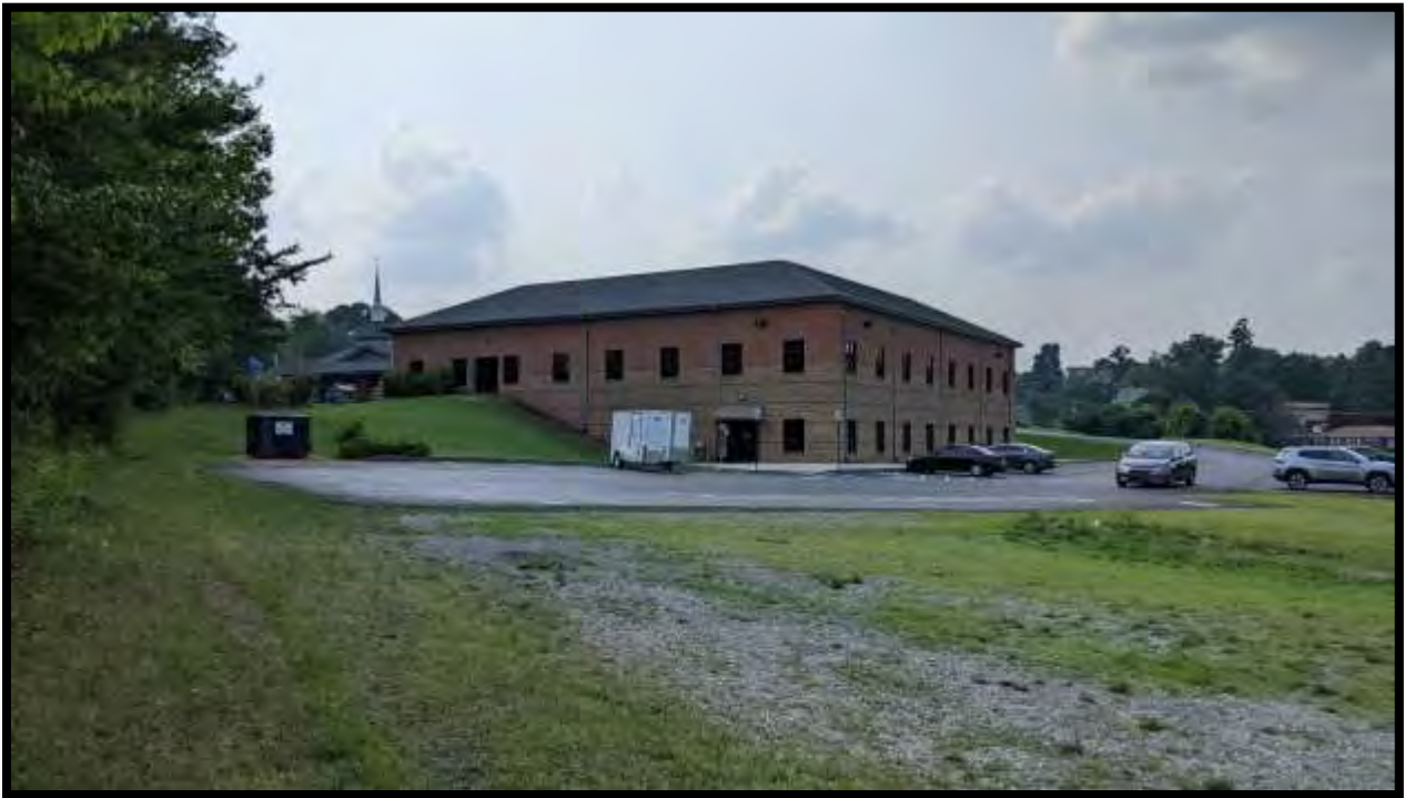
Photograph #9: South view of property North of the site.
