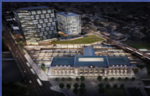
$150M+ Investment by Amtrak into Penn Station
