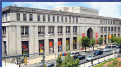
$115M Renovation of the Enoch Pratt Library Downtown
