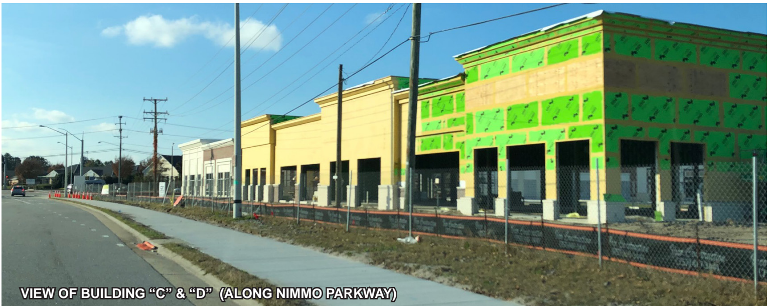
VIEW OF BUILDING "C" (ALONG NIMMO PARKWAY)
