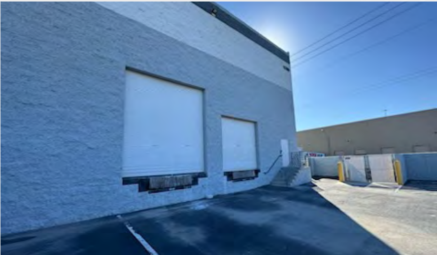
Exterior - Dock Doors
