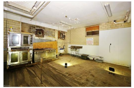
Lower level kitchen
