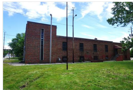
W. side of building
