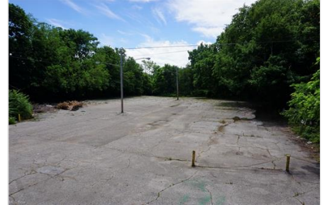
Huge rear parking lot.
