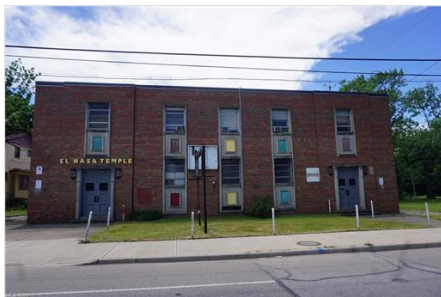
Solid brick building
