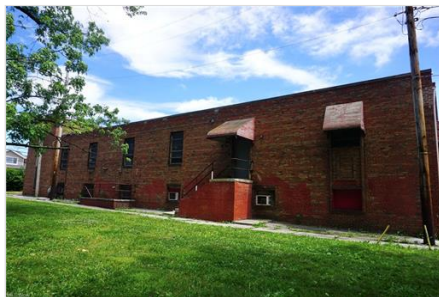
W. Side of building
