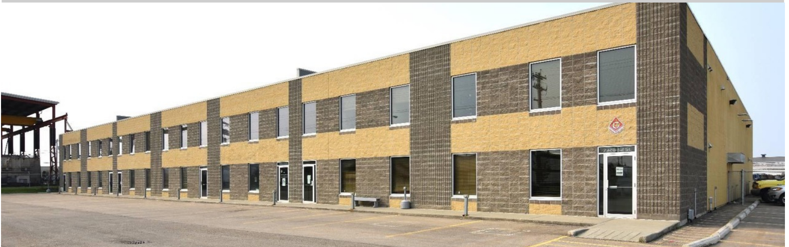
7304/28 - 52st, Edmonton 35,728sf on 2.3 acres 2000A/600V Heavy Power - $7.2m
