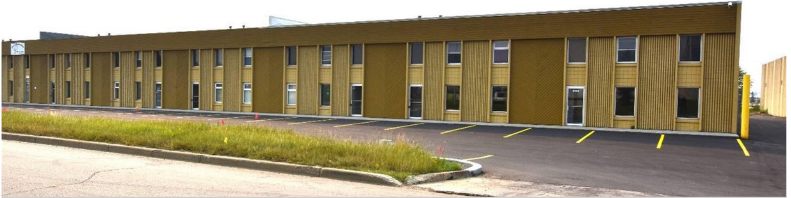
2101 - 84th Ave. Sherwood Park 39,060 sf on 3.53 acres 2000A/600V Heavy Power - $7.2m
