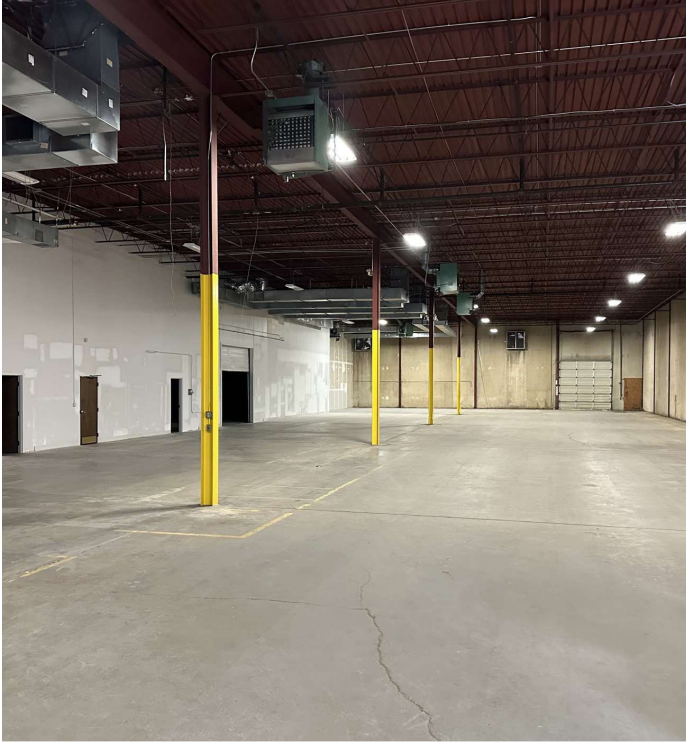
Newly Painted Wall
