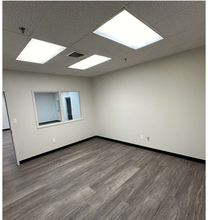
Renovated Office with New Paint + LVT
