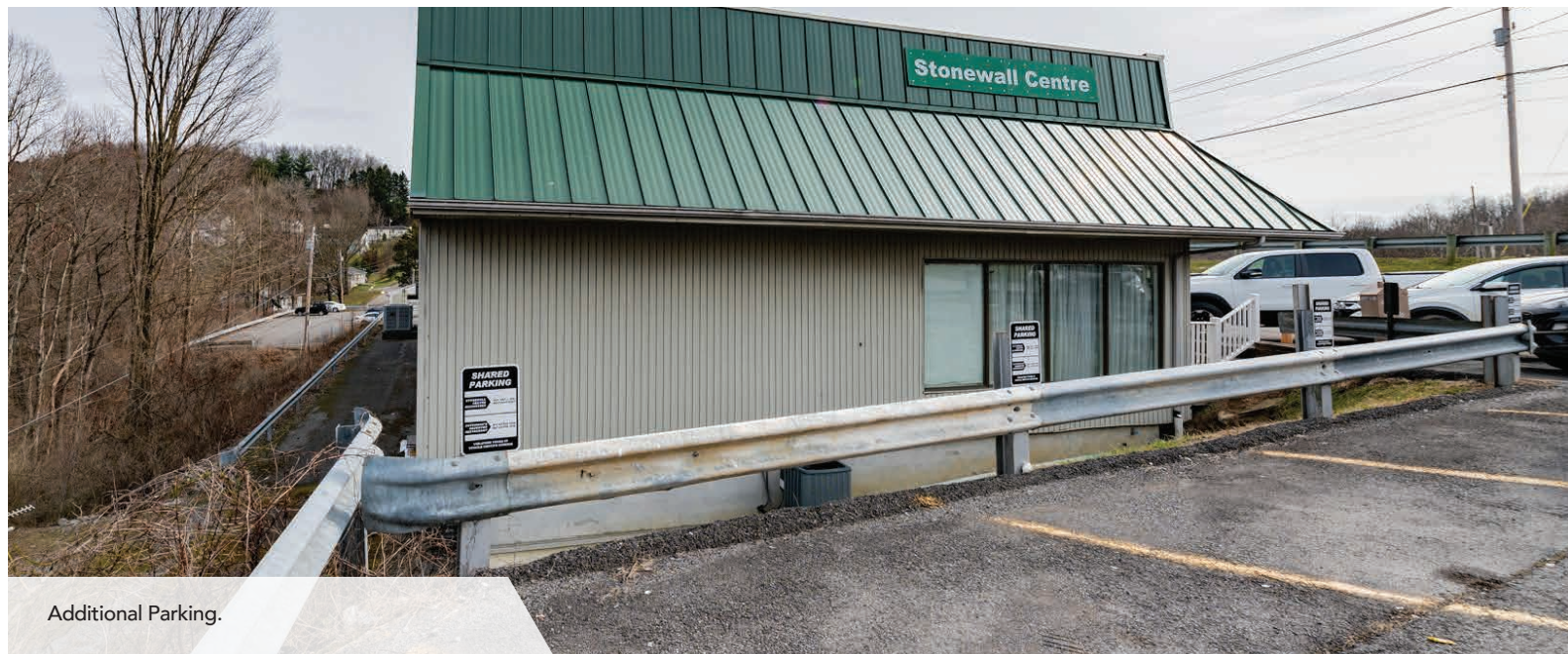
Front Exterior/Entrance to Suite.
