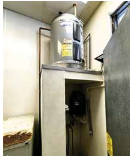
38-Gallon Electric Hot Water Heater/Mop Sink
