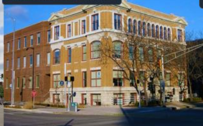
303 North Alabama Street
