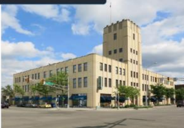
333 North Alabama Street
