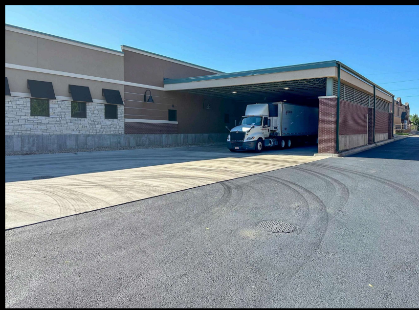
2 Covered Loading Docks - View 1
