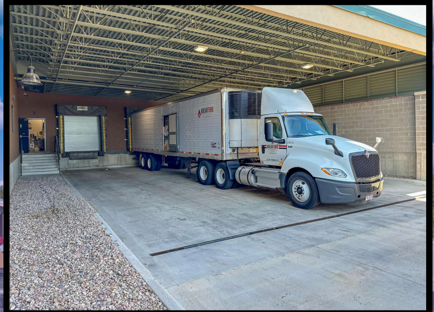
2 Covered Loading Docks - View 2
