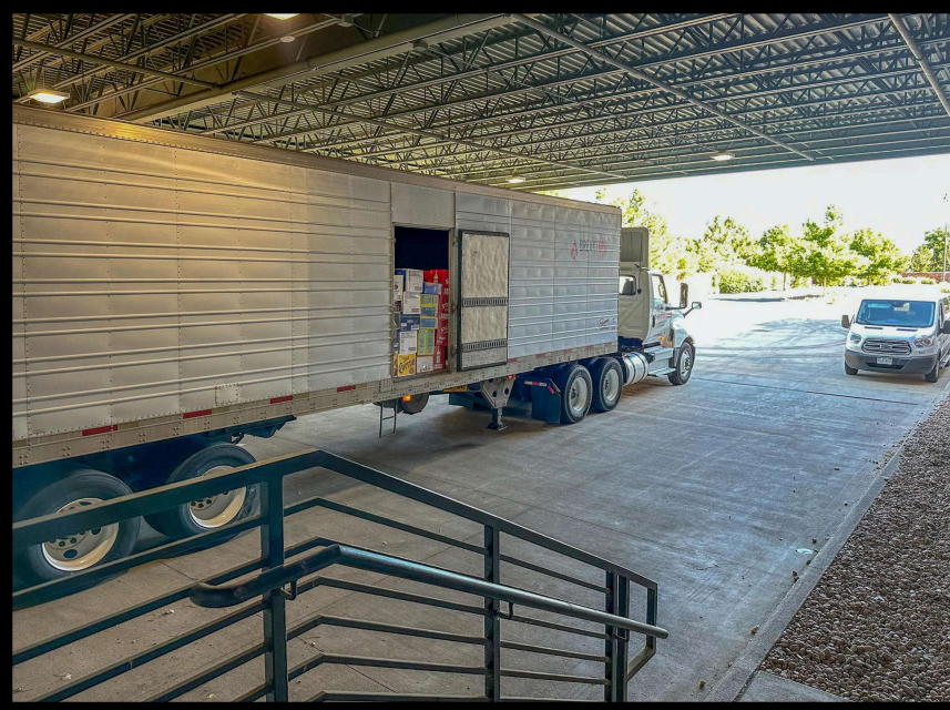
2 Covered Loading Docks - View 3
