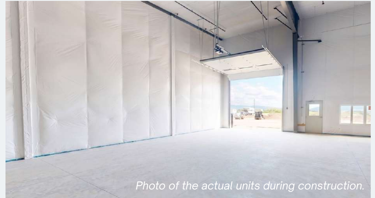
Photo of the actual units during construction.
