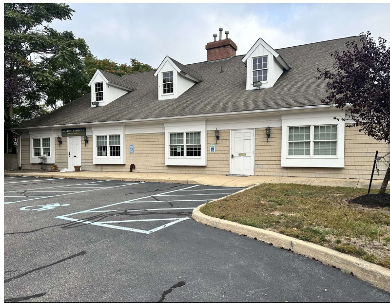
36 Rte. 25 A | ADA Parking in Rear
