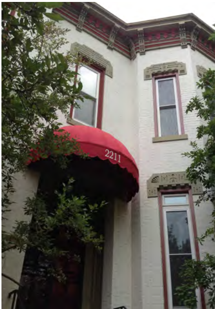
4. Italianate style rowhouse on Glenarm Pl. Note the heavy roof cornice, elaborate window headers, and tall narrow windows.
