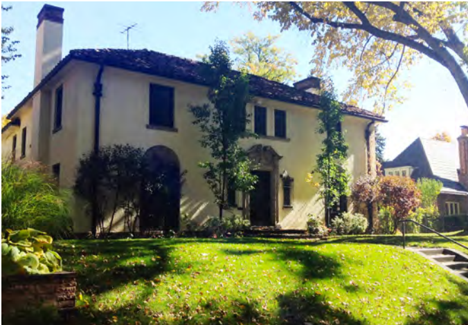
4. This Mediterranean Revival style structure has a stucco façade, a low-pitched barrel tile clay roof, and a central entry with decorative pediment, symmetrical window bays, and multiple chimneys.
