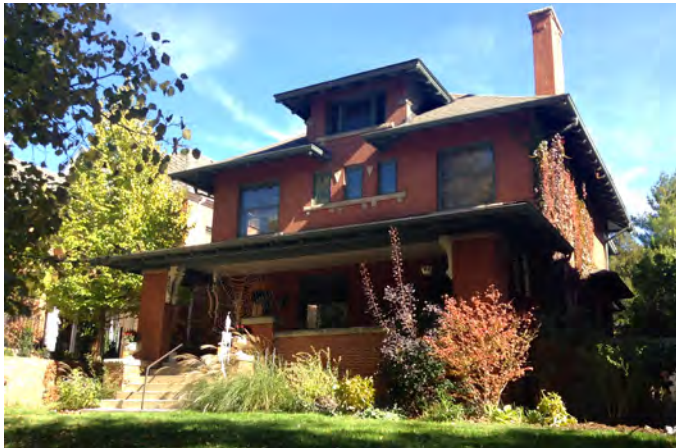
3. The Denver Square style residence with Craftsman ornamentation illustrates the boxy massing and the common red brick construction found throughout the district. While generally they have central entrances and no porches, note the full width porch and offset entry.
