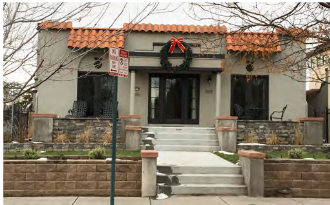
5. Mission-Revival style house with clay barrel tile roof accents.
