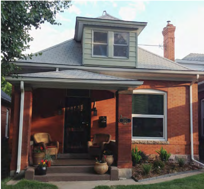
3. Simplified Classic Cottage. Note the masonry porch piers, the large overhanging roof eave, the dormer window in the hipped roof, and the jack-arch window
