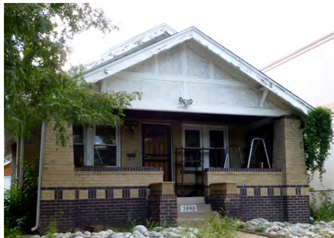
6. A small 20th century Bungalow with Craftsman detailing, including tapered brick porch columns and railings, and half-timbering details in front gable end. Note the paired windows on the front of the home.
