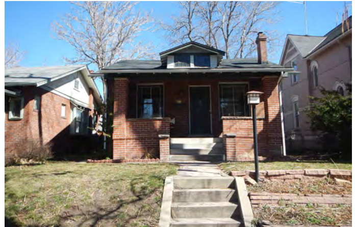
10. Bungalow with a full-width porch under the main roof, and a multi-light dormer. Note the central steps and walkway leading in a straight path to the front entry.
