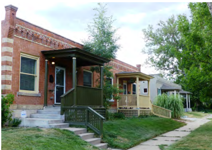
5. Red brick rowhouse with corbelled roof detailing and raised columns at roof parapet. Note steps leading from the sidewalk into the front lawn to accommodate the Denver Hill.
