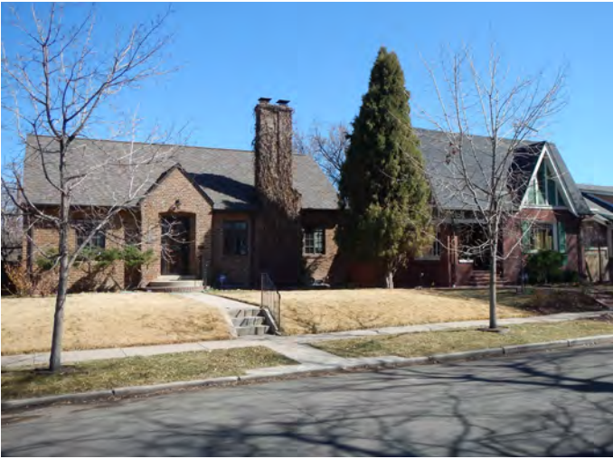
1. Streetscape fronting onto Alamo Placita Park. Note the open front lawns with the Denver Hill, and the Tudor style architecture typical of the later development of the neighborhood.
