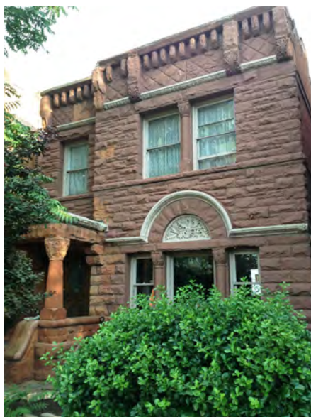
4. Romanesque style building on Stonemen's Row. Note the masonry façade, the Romanesque style column capitals, the semi-circle arch motif over a Palladian-esque window motif, and the heavy cornice.
