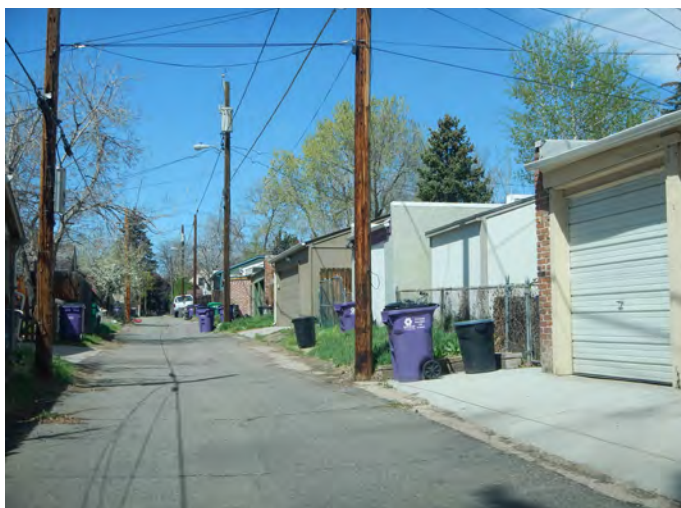
8. Typical alleyway. Note the low one-story masonry garages with single bays, the flat roofs concealed by parapet walls and the orientation of the structure at the rear of the lot.
