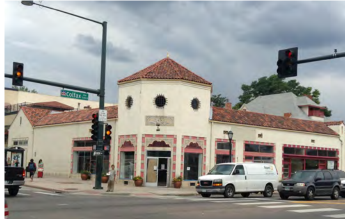
8. Commercial development on Colfax in the Spanish Revival Style. It is one-story high, has symmetrical massing, large display windows with transoms, and a barrel clay tile roof.
