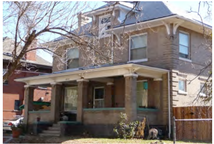
4. Craftsman Denver Square. Note the more decorative features and details, including front dormer window, broad overhanging roof eaves supported by brackets, corner brick quoins, and corbelled masonry piers supporting a full-width bracketed porch.
