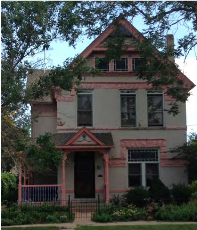
6. Typical Eastlake influenced structure within the district. Note the gable front with decorative bargeboards, wrap around one-story porch, elaborate leaded glass windows, tall chimneystack, and decorative stone banding.
