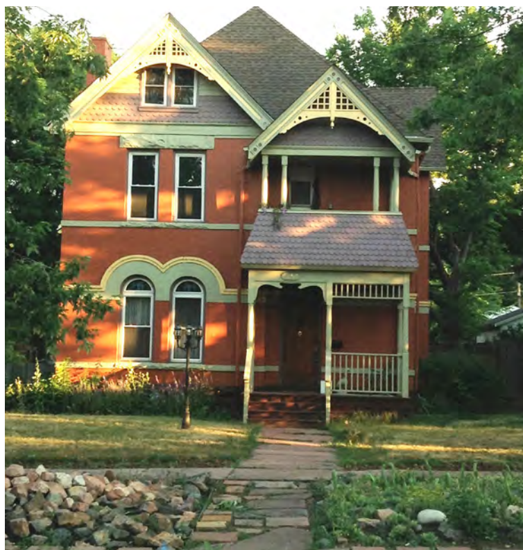
11. Typical two-story Queen Anne residence with open front yard and front sandstone walkway leading from sidewalk to front porch and door.
