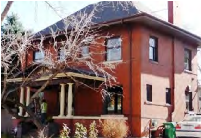
3. Vernacular Classical Revival Denver Square. Note the relatively austere brick building with hipped roof, symmetrical placed windows, stone window sills, diamond pane windows, and classical Doric porch columns providing architectural relief.
