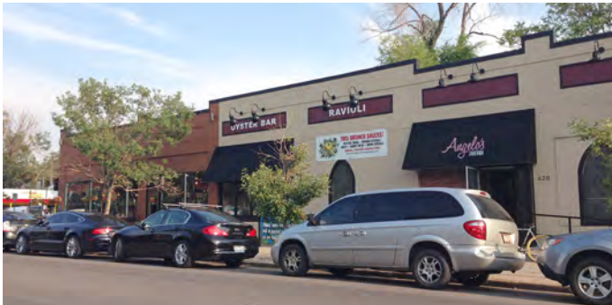
3. Several early 20th century commercial buildings are located on the south side of 6th Avenue with boxy, symmetrical massing.
