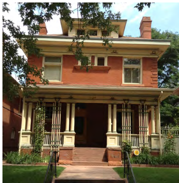
4. Typical Denver Square with Classical Revival elements. Note the classical wood columns supported on a pedestal at the full-width porch, and the corner masonry quoins.
