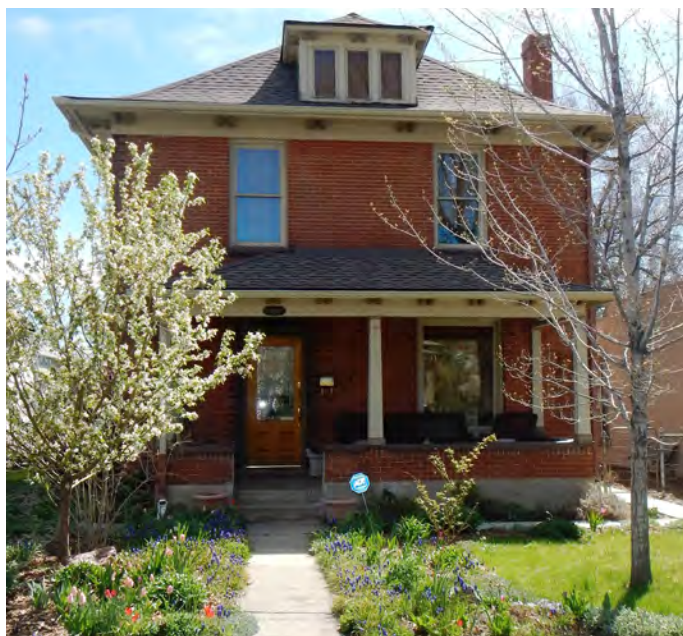
7. At-grade walkway leading in a straight path from the curb to the slightly off-set entry door to this Denver Square with Classical Revival elements. Note the dormer in the roof line and the classical Doric columns and the symmetry of the façade.
