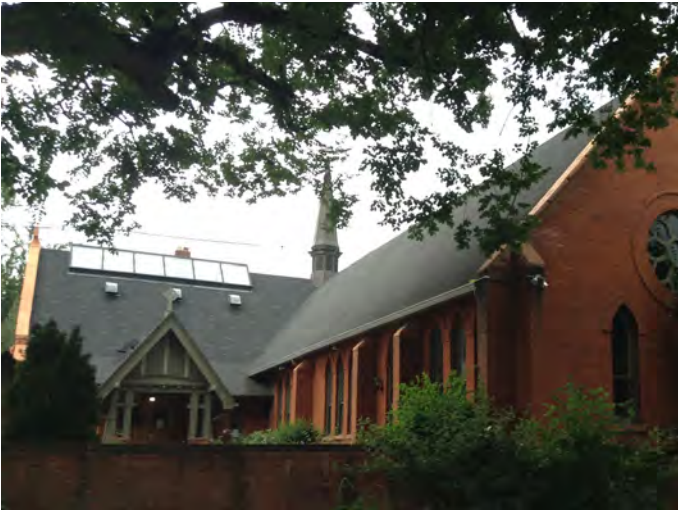
9. St. Barnabas Episcopal Church was designed in the Gothic Revival Style. Religious buildings are typically located at corners on east-west streets.
