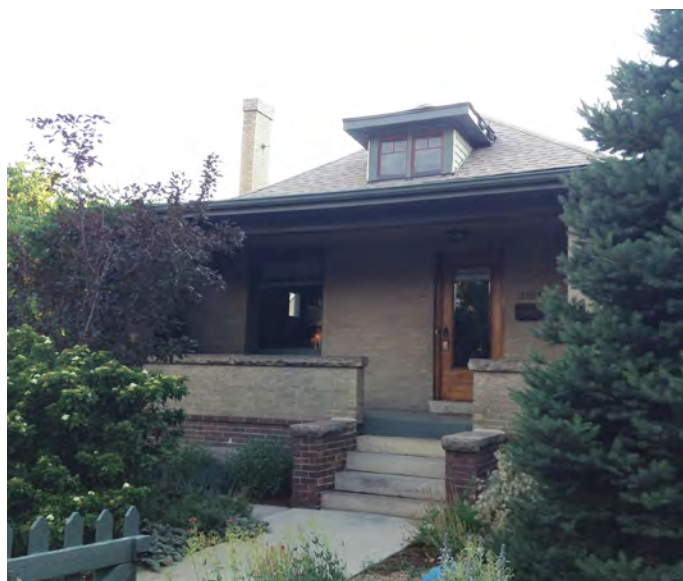
4. Craftsman Bungalow. Note the masonry porch, the dormer window in the hipped roof, and the overall simple ornamentation.
