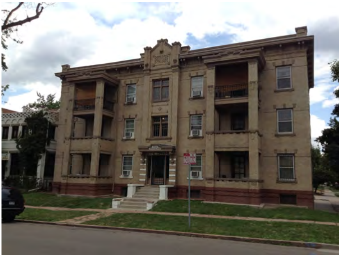
11. Turn-of-the-century apartment development with projecting, symmetrical balconies. Note the sandstone sidewalk with a few steps leading to the front door to accommodate the front yard slope.
