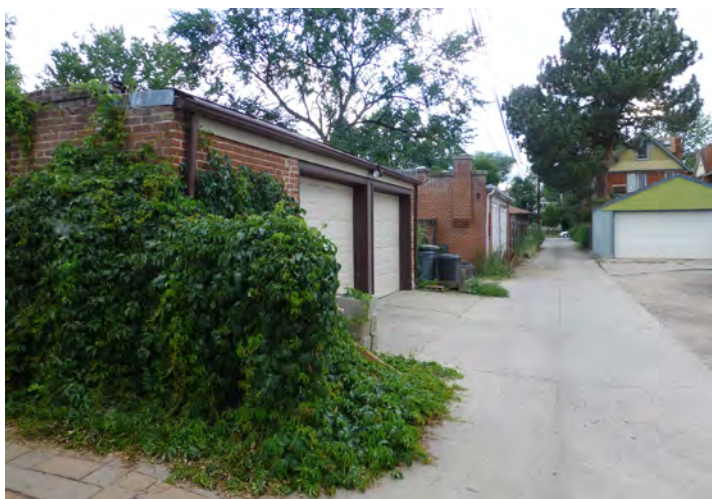
12. Partial view of carriage lot on right from alley. Note the typical one-story rectangular shaped brick garages.
