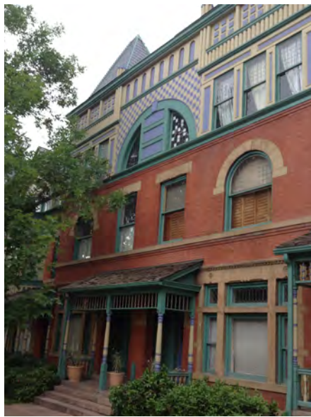
5. Queen Anne rowhouse on 21st Street. Note the historic sandstone sidewalk, brick construction with stone foundation, steeply pitched slate roof, and the one story porches with fretwork and spindle columns.
