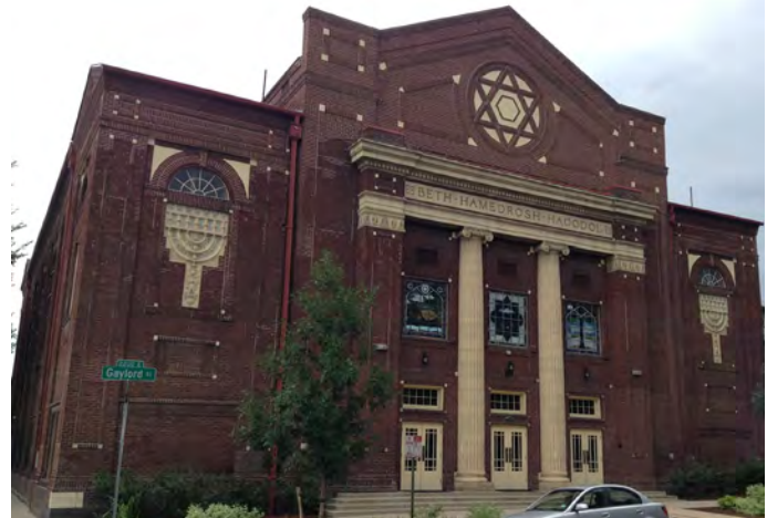
10. Beth HaMedrosh Hagodol was a Jewish synagogue in the Classical Revival Style that has been converted to a Christian church. Note the building's symmetrical massing, prominent entrance, brick façade and terra-cotta ornament.
