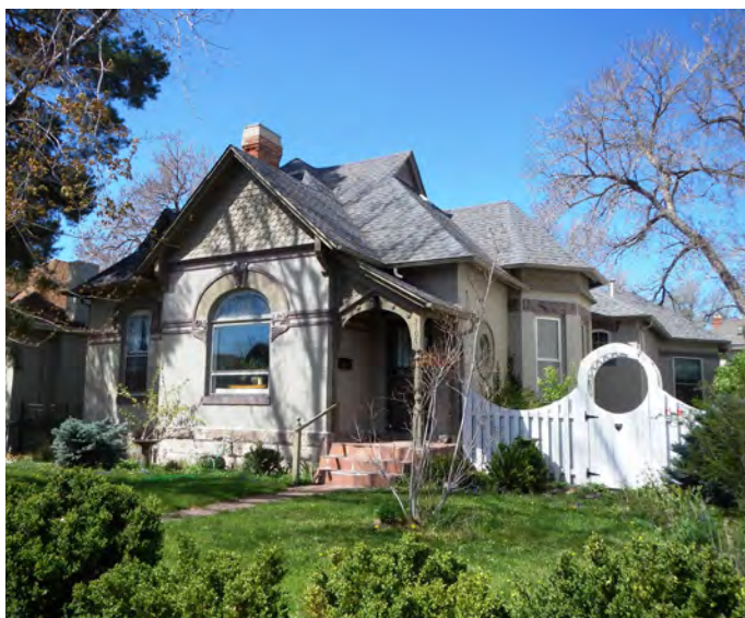
3. Queen Anne style cottage. Note the complex roof form, the fish scale shingles, the stone foundation, the decorative banding, the arched window with semi-circle brick arch above, and the spindle column on the covered stoop entry.
