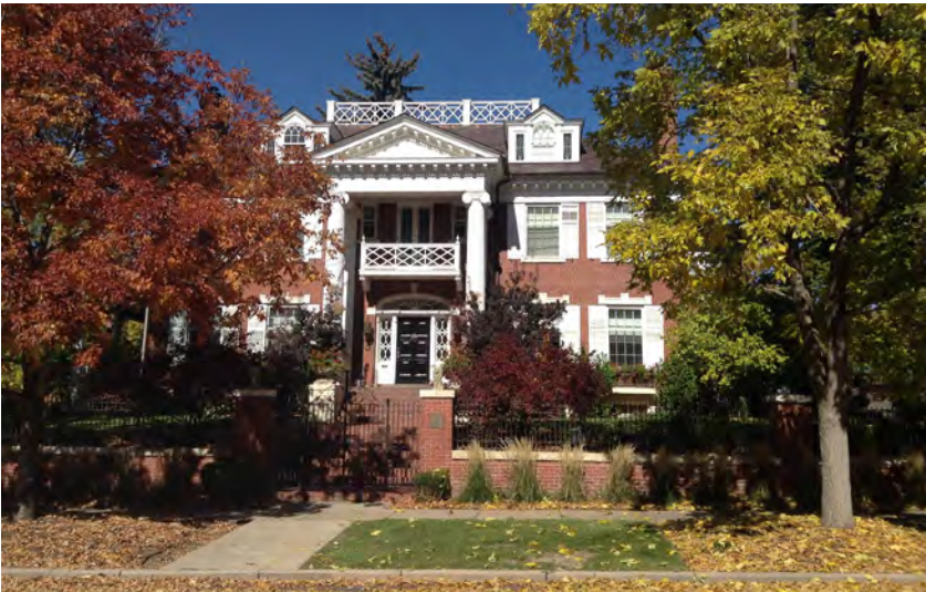
7. The Classic Revival style structure with a large central walkway to the portico entry is typical. Note the historic fenced in front yard with masonry foundation, concrete coping, and iron fence above.
