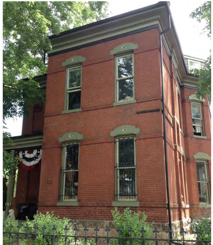
7. Typical brick Italianate structure within the district. Note the decorative cornice, the tall narrow windows with elaborate stone window headers and sills, the low pitched roof, rectangular projecting forward bay and stone foundation.
