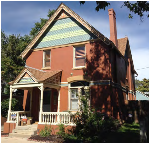
6. Typical Queen Anne development within the district. Note the forward facing gable with fish-scale shingles and decorative sunburst and barge board, the projecting front porch with cross gable roof with a matching fish scale shingles and sunburst motif, and the arched ground-floor window.
