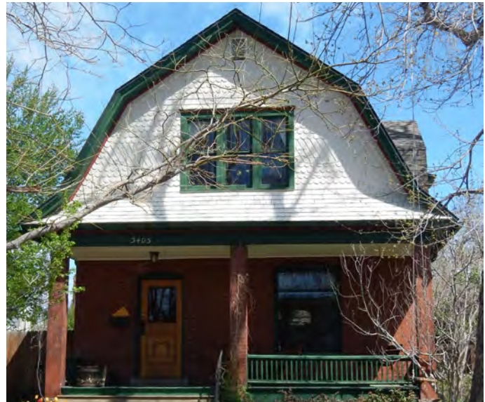
6. Queen Anne style structure with a forward facing gambrel roof. Note the masonry porch columns, the triple window bay, and fish-scale shingles in the gable.
