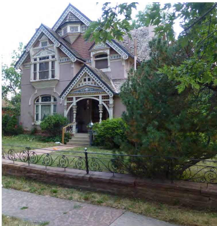
10. A few high style Queen Anne residences are found in the district, such as the Frederic Neef House (individual Denver Landmark). Note the more complex roof shape and ornamentation, and elaborate window decoration and arched porch opening. The house has a low masonry retaining wall.
