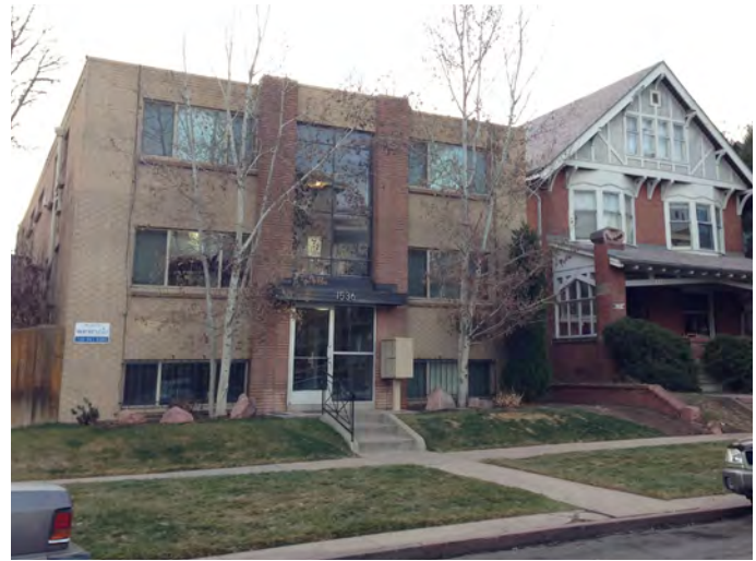
6. Mid-century apartment buildings are generally two to four stories high and have simplified forms and ornament. They usually do not have porches or balconies.
