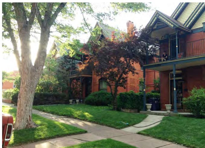
2. Streetscape on the north side of the district with Queen Anne Style buildings. Note the uniform setback and the large front yard, when compared to the front yards on Stonemen's row.
