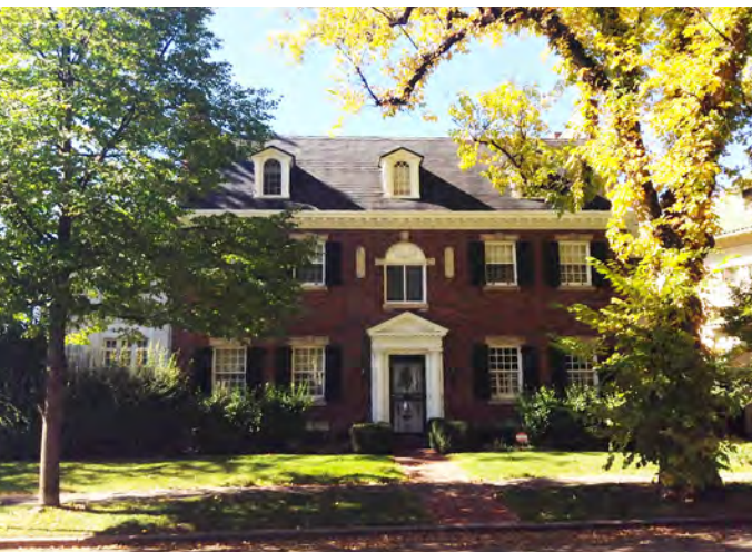
5. This Classical Revival style structure has the typical red brick construction, symmetrical façade, triangular pediment surrounding the central entry, and dormer windows in the gable roof.
