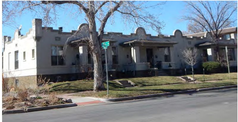
7. Duplex structures in the Mission Revival style. Note the stepped parapet and the decorative corner tower at parapet that serves as the overall ornamentation on this simplified, one-story structure.
