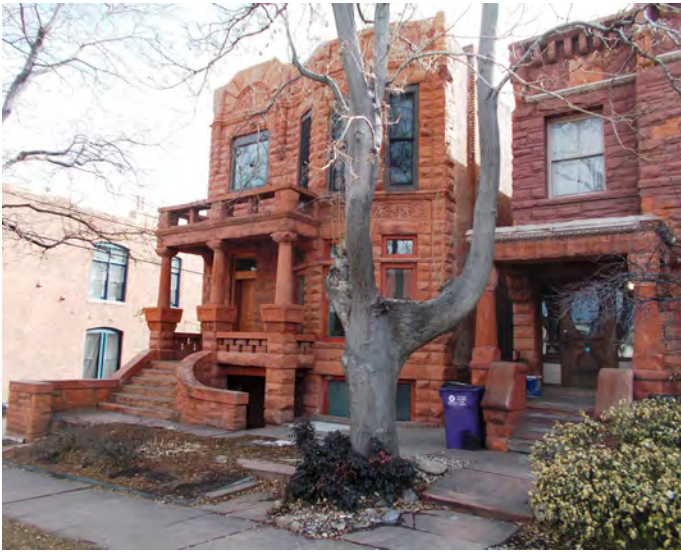
6. Streetscape of Stonemen's Row. Note the raised masonry porch forms on both these structures, with heavy Romanesque columns and detailing, the wingwalls and the second-story balcony on the structure in the background and the one-story configuration of the porch in the foreground.
