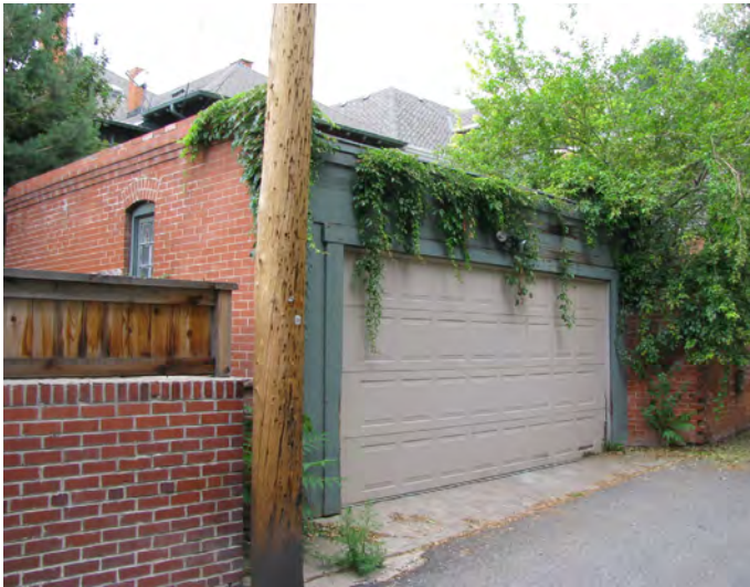
8. This detached garage has roof and parapet, red brick construction that matches the primary residence, and alleyway location is typical.
