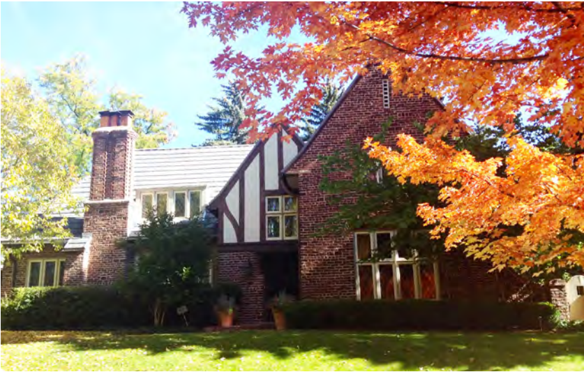
6. Note the asymmetrical massing with an offset entry, the red brick construction with stucco and timber framing accents, the decorative chimney, and the leaded glass casement windows on the Tudor Style structure.
