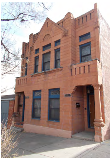
3. Romanesque style building on Stonemen's Row. Note the masonry façade, tall narrow windows, and the semi-circle arch motif in the building parapet.
