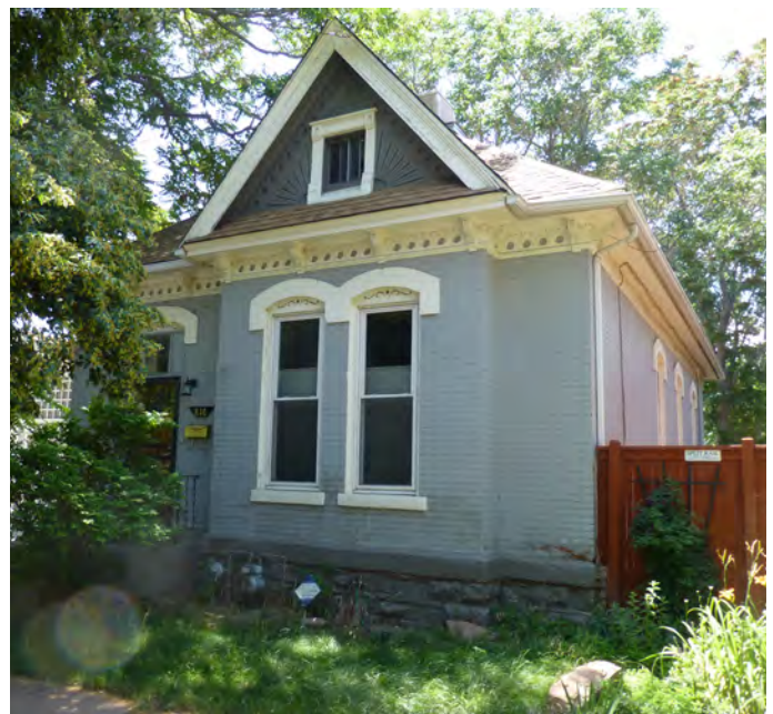
9. One-story Queen Anne Cottage within the district. Note the raised stone foundation, the paired window bays with arched brick headers, the decorative cornice and brackets and the forward facing gable with a sunburst motif.
