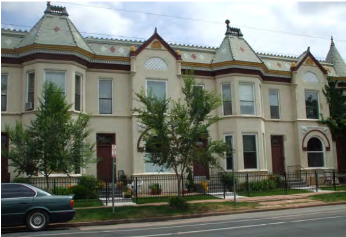
4. Multi-family Victorian eclectic dwelling fronting onto a primary street. Note this repeating projecting towers, the arched windows on the first floor with decorative headers, the transoms above the single entry door, and the decorative pattern roof.
