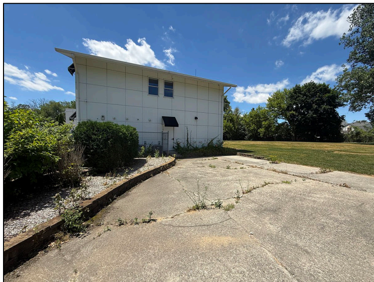
Patio area – east elevation
