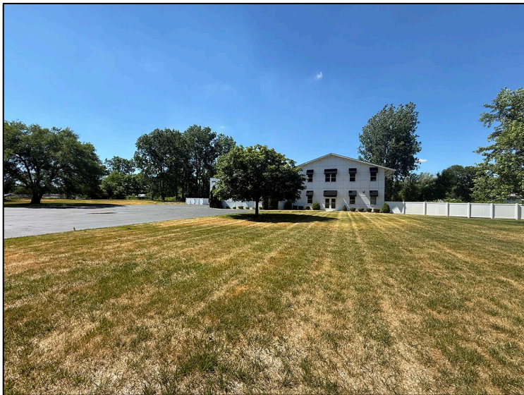
Airport Hwy view – south elevation
