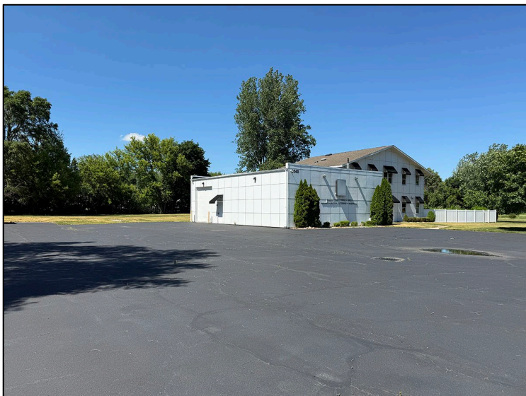
Overhead door access – west elevation
