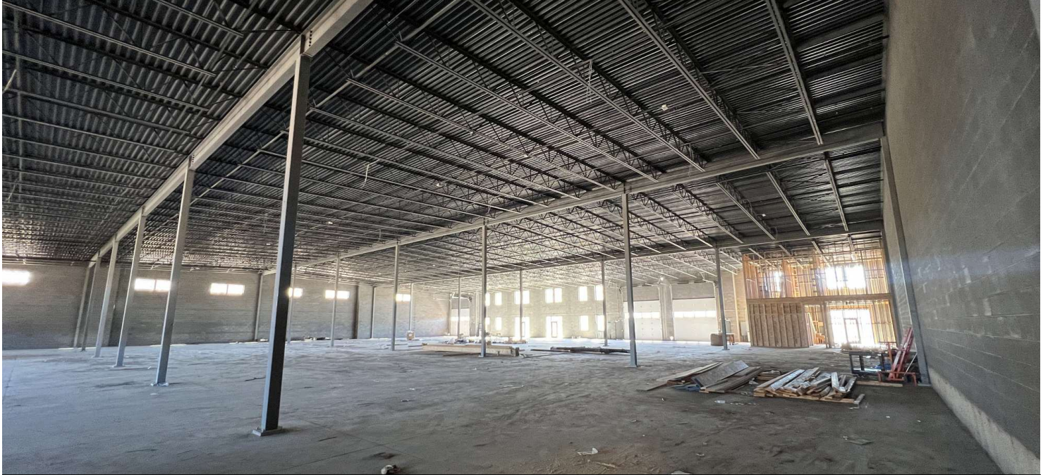
Warehouse Unit F,G,M & N
