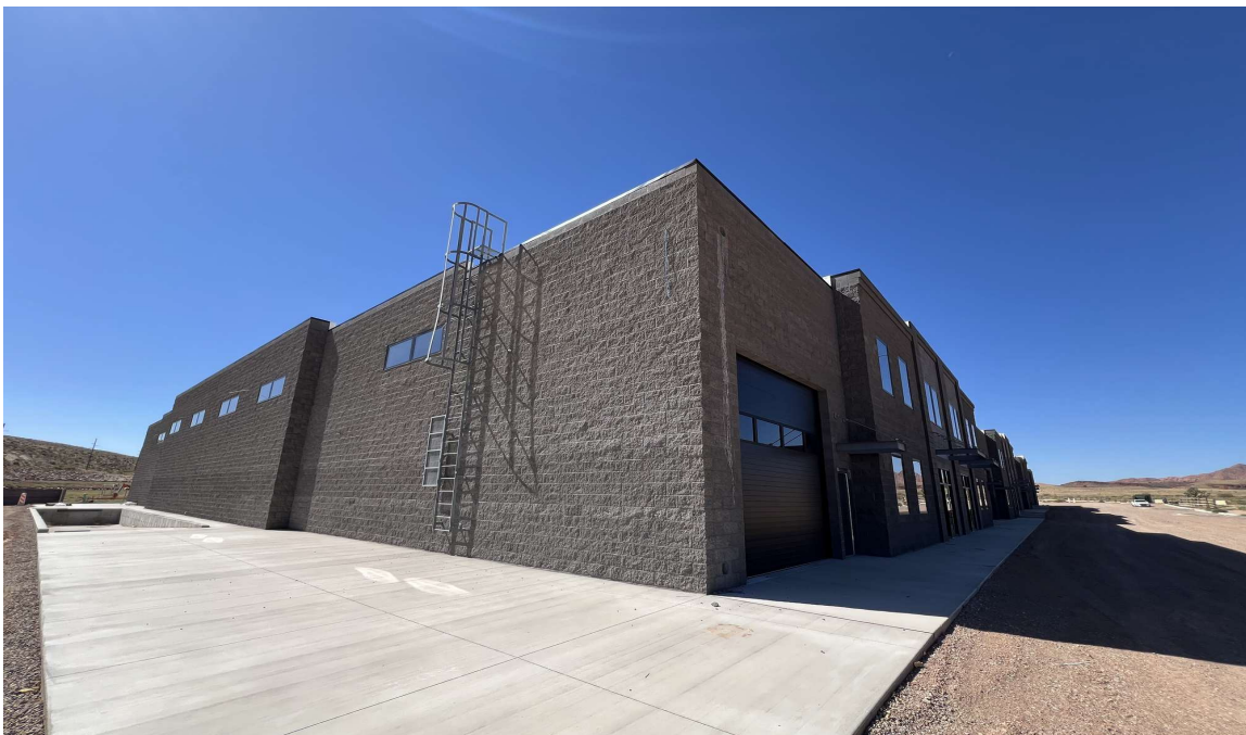
North East Corner with Loading Dock
