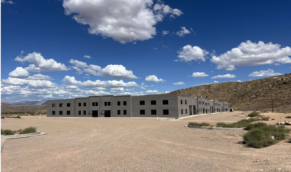
View From I-15 (South West Corner)
