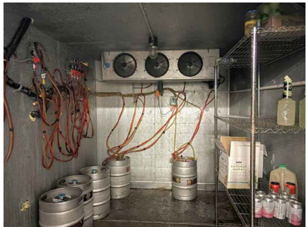
Lower Level - Walk-In Cooler
