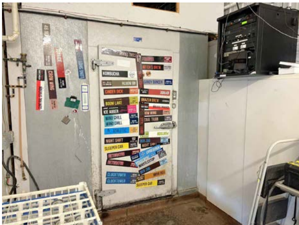
Lower Level - Walk-In Cooler
