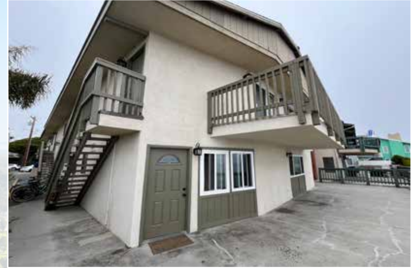
Rear and Side Exterior, 2nd Story View Balcony
