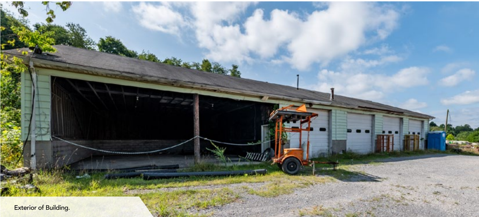
Exterior of Building.
