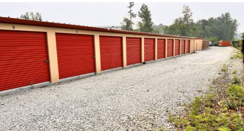
South lot building
