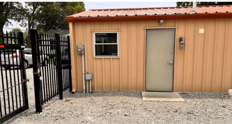
Office side door
