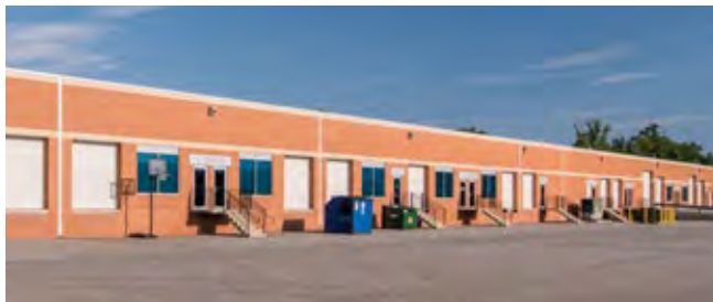
Flex/R&D dock and drive-in loading
