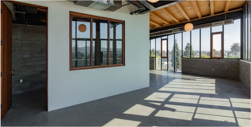
B— OFFICE INTERIOR
