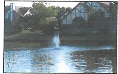
Detention pond with aerator.
