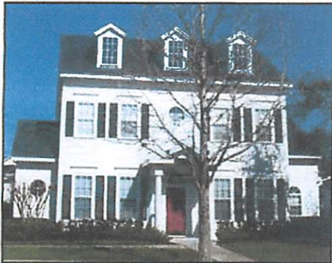
Elevation with shutters.
