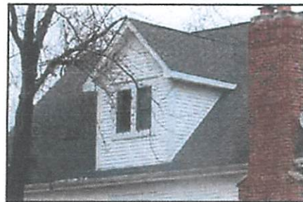
Example dormer on local home elevation .
