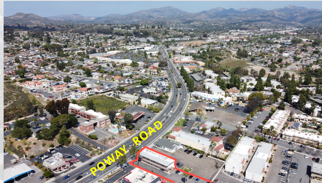
View from above the building facing Northeast.
