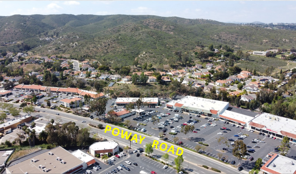
View from above the building facing Northwest.
