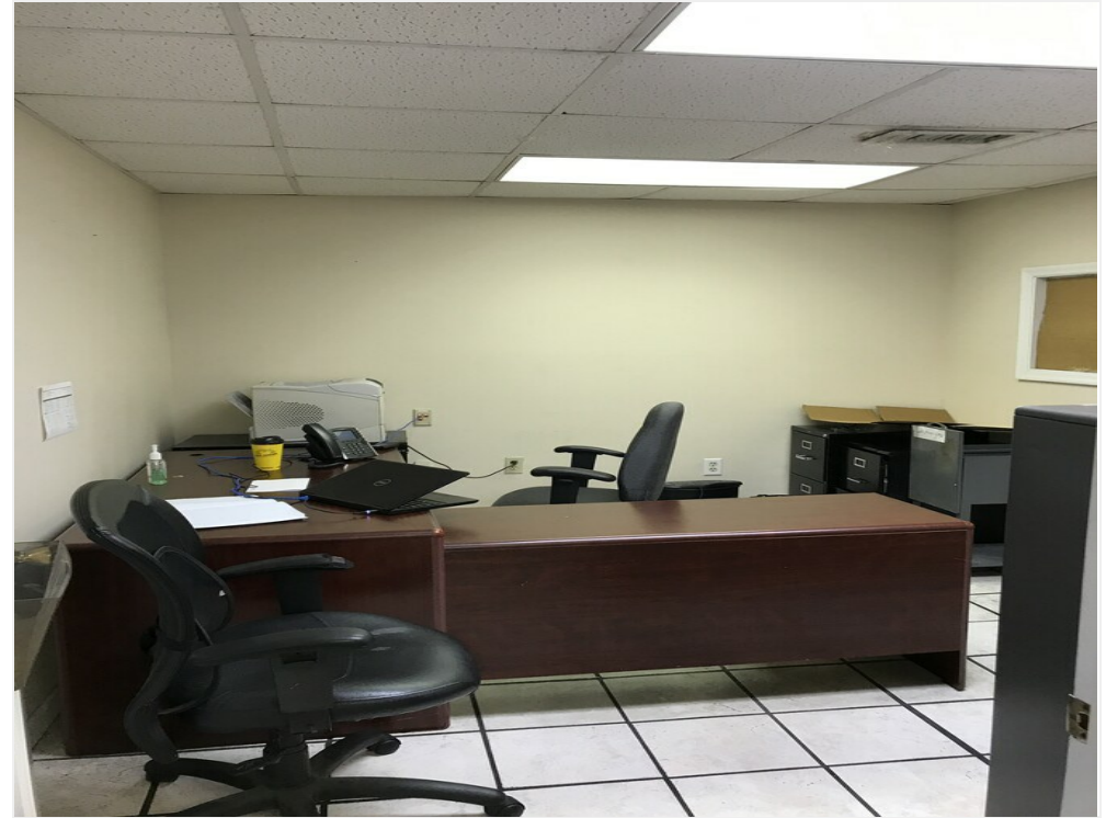
Interior Photo before refurbishment
