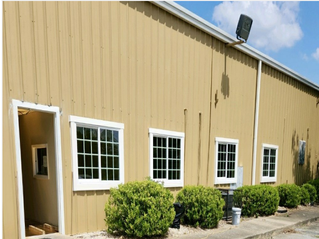
New windows progress
