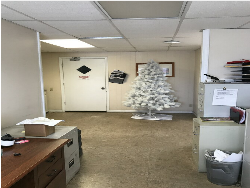
Interior Photo before refurbishment
