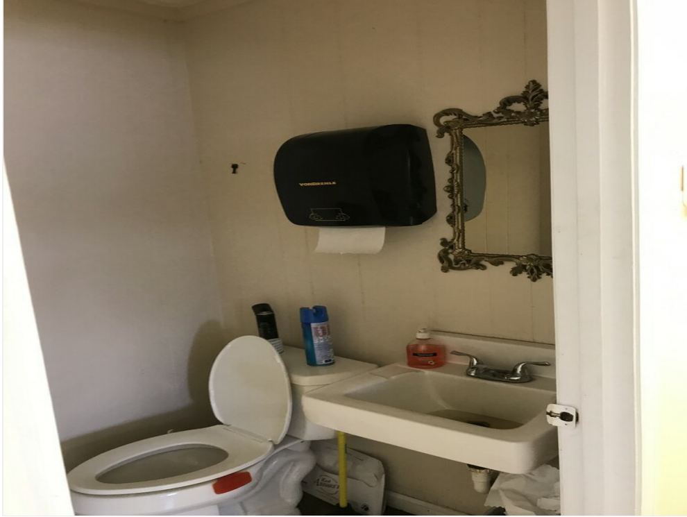
Interior Photo before refurbishment
