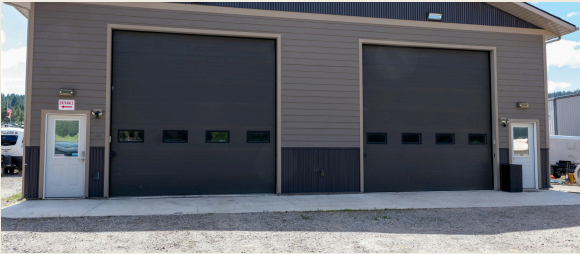
SHOP BAY — 16 FT CLEAR HEIGHT
