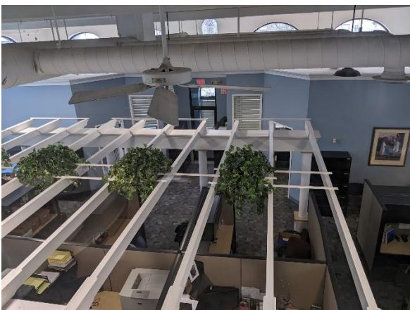
View from second floor
