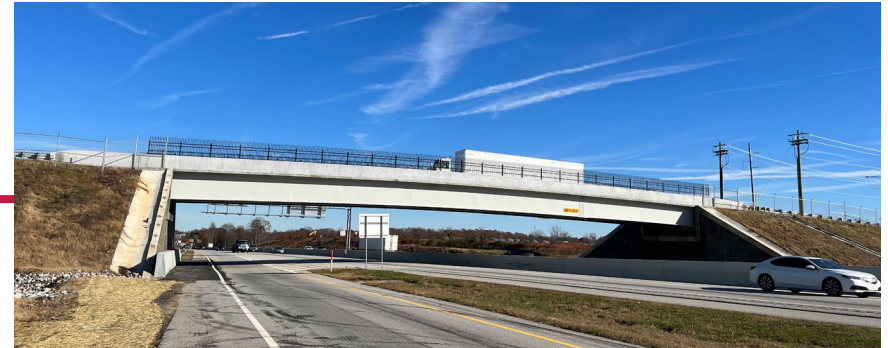
BMW PRIVATE BRIDGE OVER I-85 TO CONNECT THEIR NEW BUILDING TO THEIR MANUFACTURING PLANT
