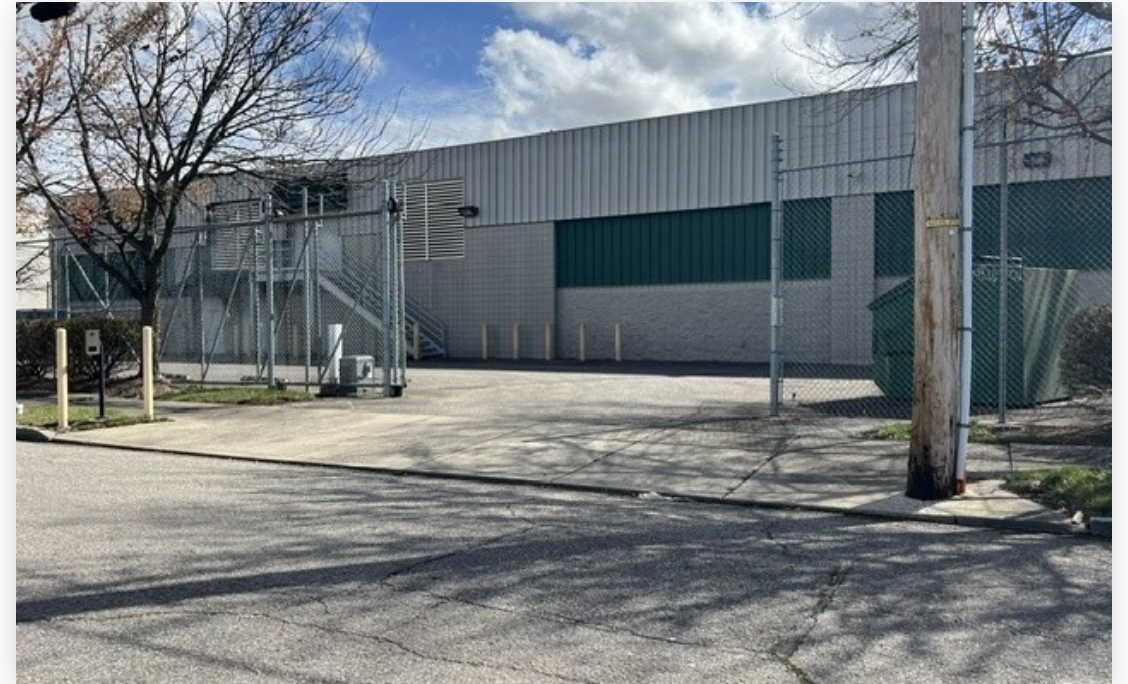
Site view: perimeter fencing and gated access
