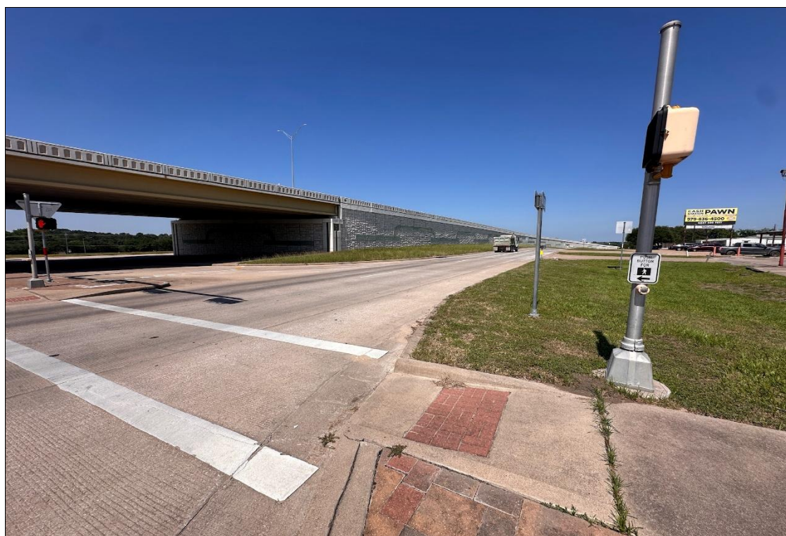
Looking east along US Highway 290 East Frontage Road with the subject property on the right
