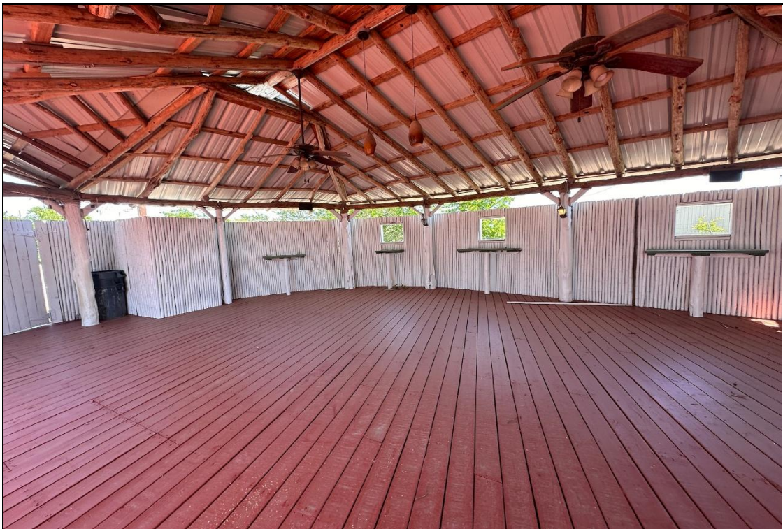
View of the patio area
