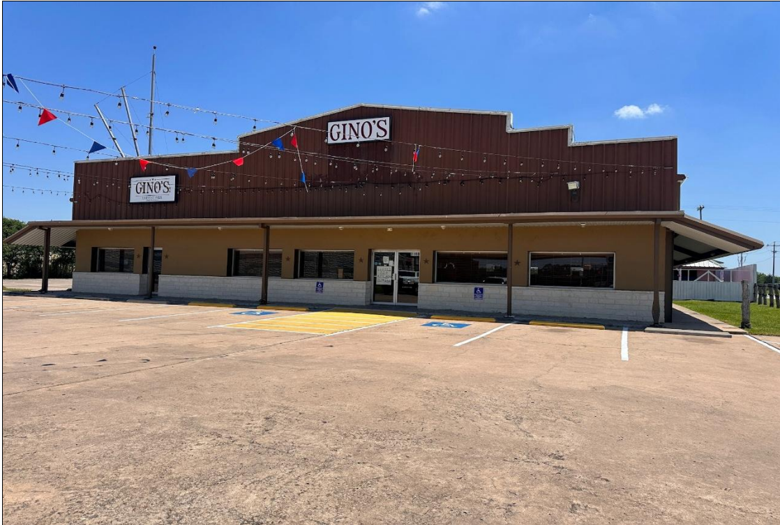
Exterior view of Building 1
