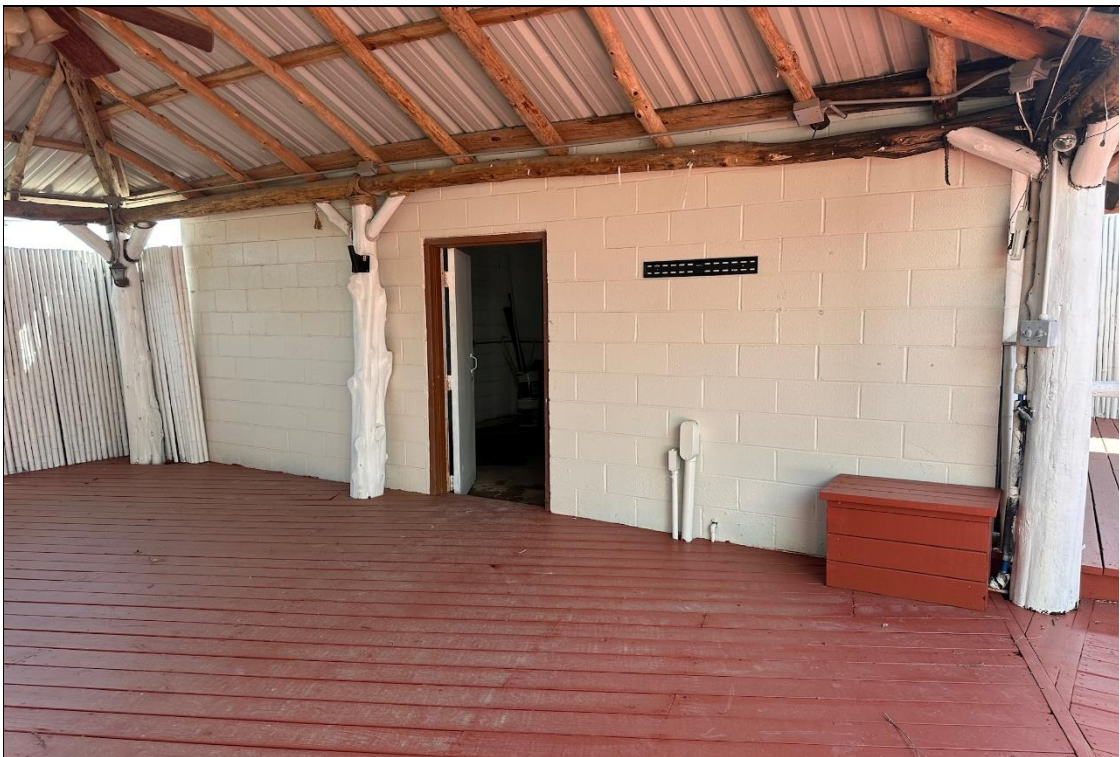
Exterior view of Building 2
