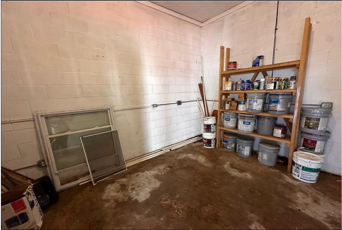
Interior view of Building 2
