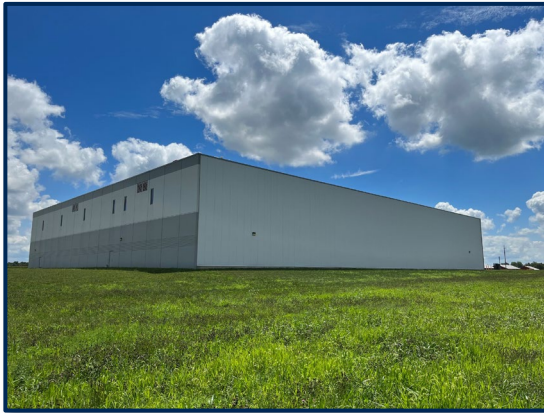
North & West Wall
