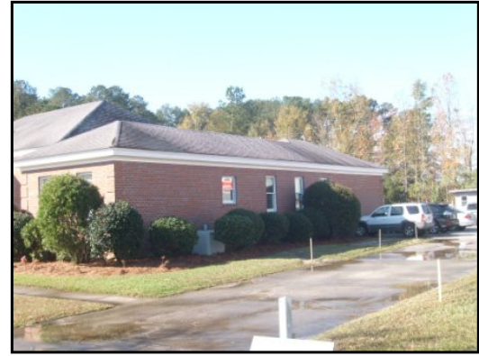
2 : Right-side elevation - facing southwest
