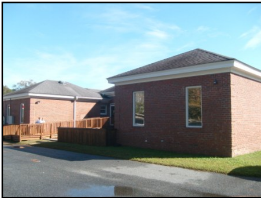
3 : Rear elevation - facing northeast
