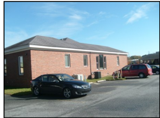
4 : Left-side elevation - facing northeast
