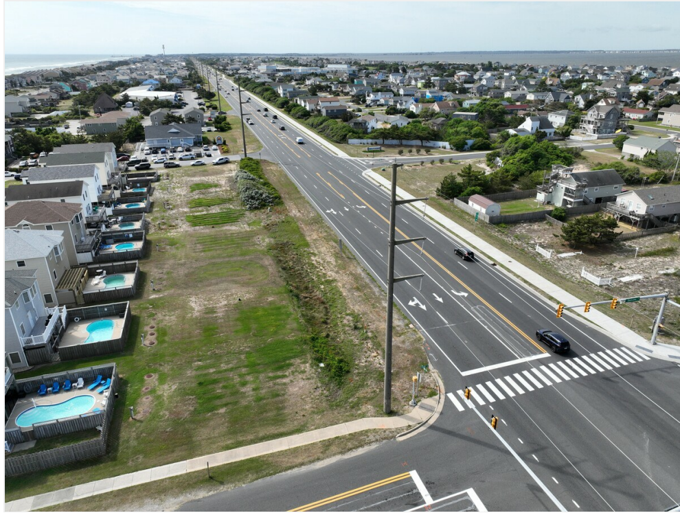
Looking South on S Croatan Hwy
