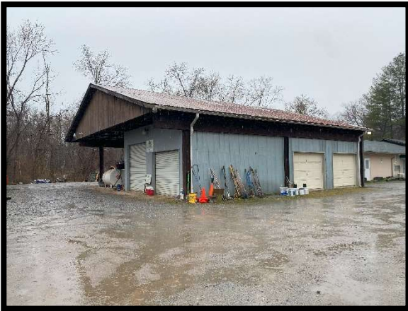
Northeast corner of the facility.
