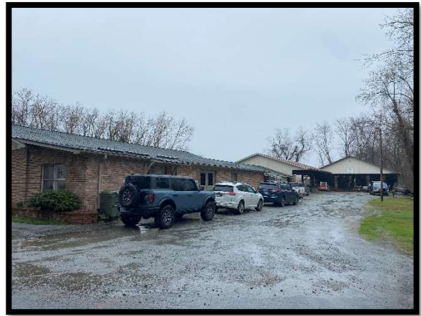
Southwest side of the facility. Note the parking area.
