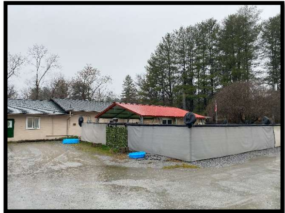
Northwest corner of the facility.
