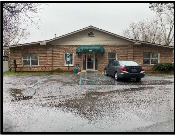
West side of the facility. Main entrance into Dogs in Suds.
