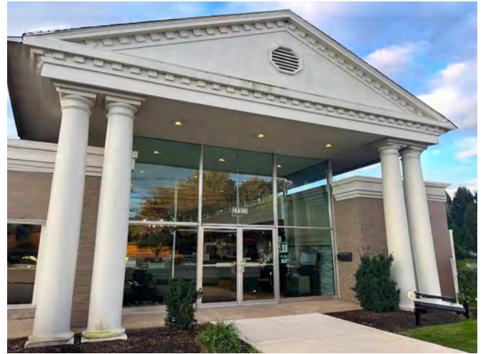
Front Entrance Outside
