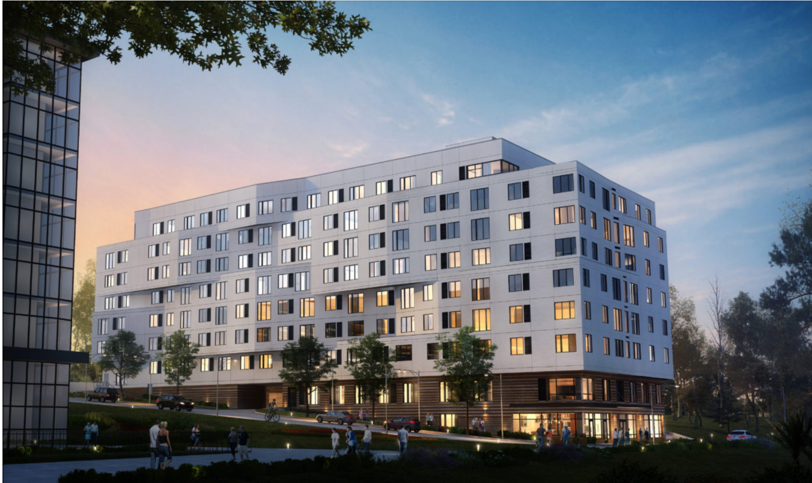
5330 W. 11 th Ave 133 Units – 120 Parking Spaces via RTD Garage – Affordable Housing Project
