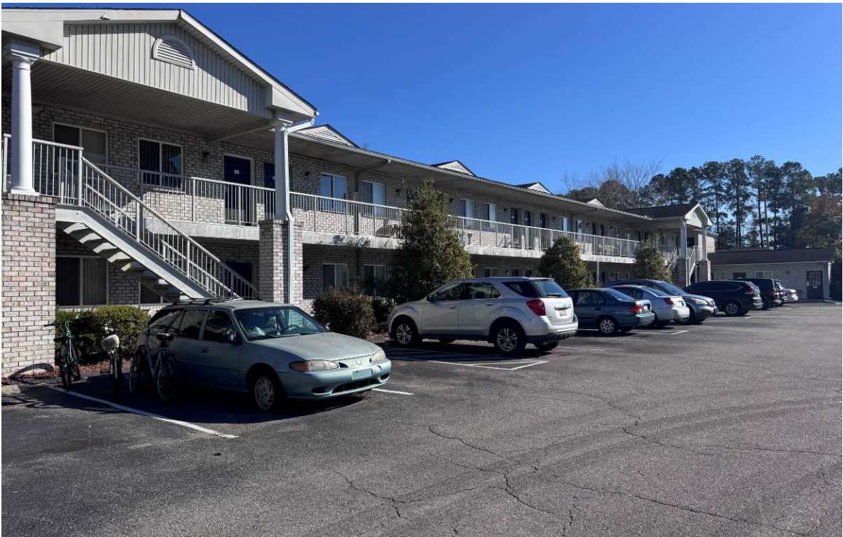
29-Unit Building with All 1-BR Units, Office, Laundry on Right Side
