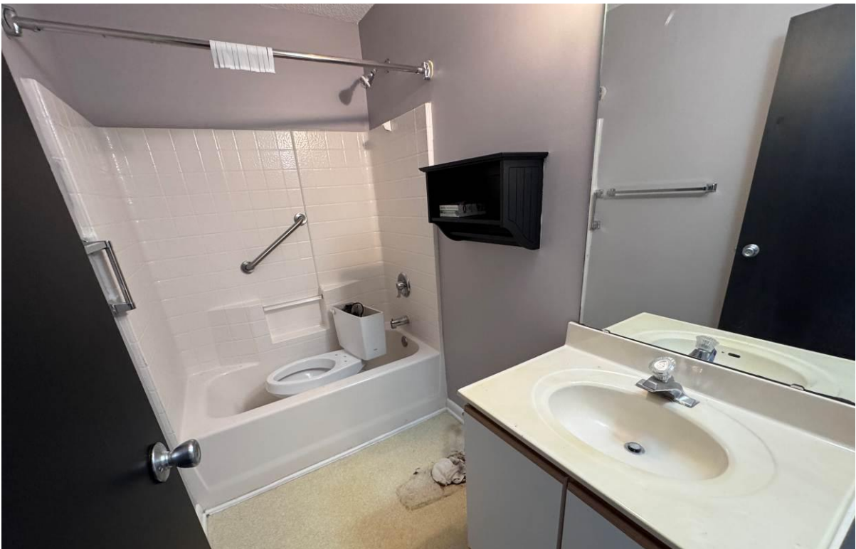
Unit 4 – Flooring Being Replaced
