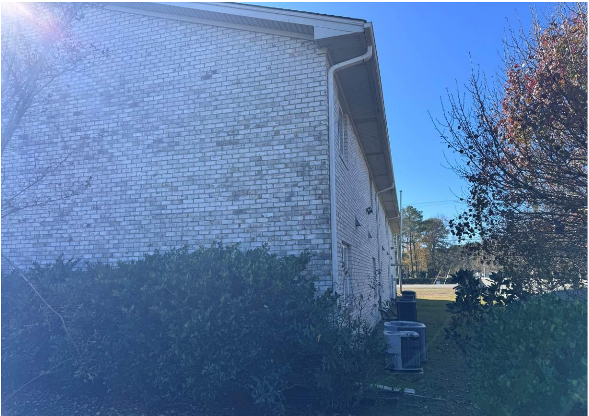
Rear and Side Exterior of Building Improvements (29-Unit Building, Above) (14-Unit Building Below)
