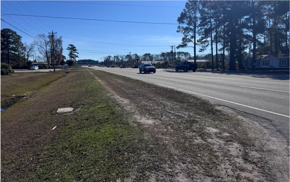
Holmestown Road Frontage – Looking East towards Highway 17 Bypass
