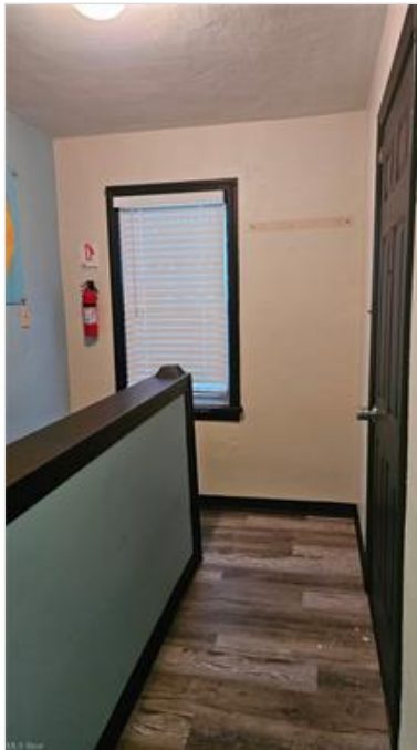
Hall with a textured ceiling and dark wood-style flooring
