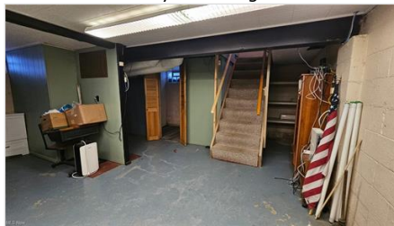
Finished basement with concrete block wall and stairway
