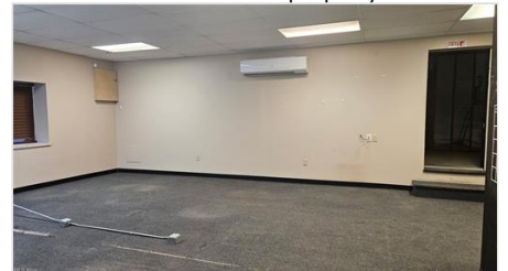
Spare room featuring a drop ceiling, a wall mounted AC, and carpet floors
