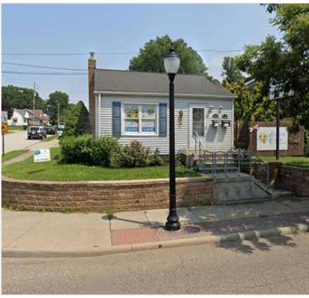
Bungalow featuring a chimney and a shingled roof
