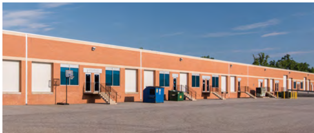
Flex/R&D dock and drive-in loading
